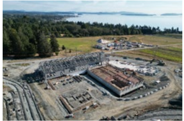
Construction at the Centre for Plant Health
