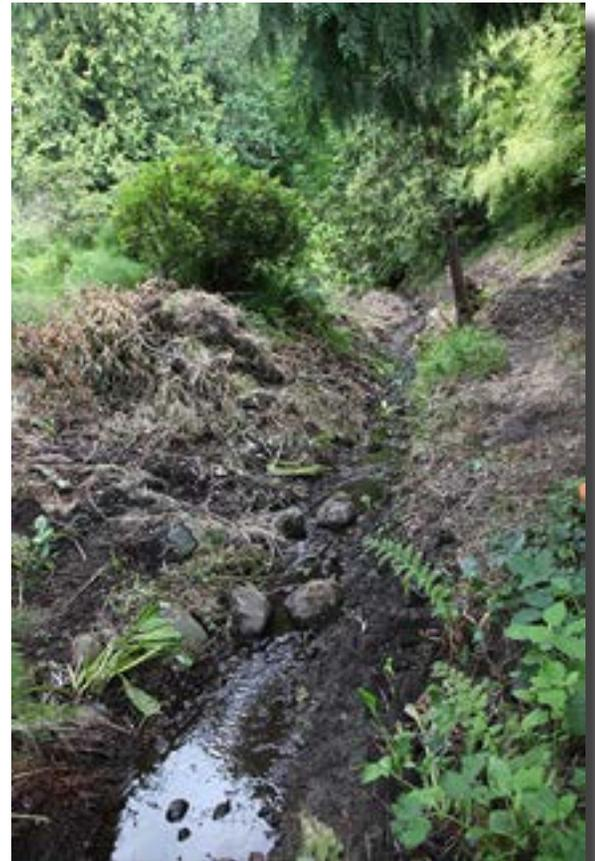
for one meter on each side for the first time in many years. Now the engineers can assess the remedial work required. For consideration are lining the streambed with rocks, adding riffles to slow the water and avoid erosion, and finally building up the lower slopes for future plantings.
