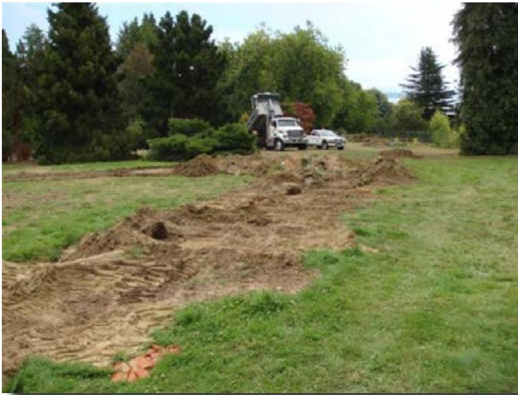
North Saanich Parks made it a priority and tackled the job in late summer. Trenches were dug so the water supply could be studied to determine where it originated, the amounts and that it was clean. There are aged drainage and irrigation systems throughout the Park with collapsing clay tiles.
